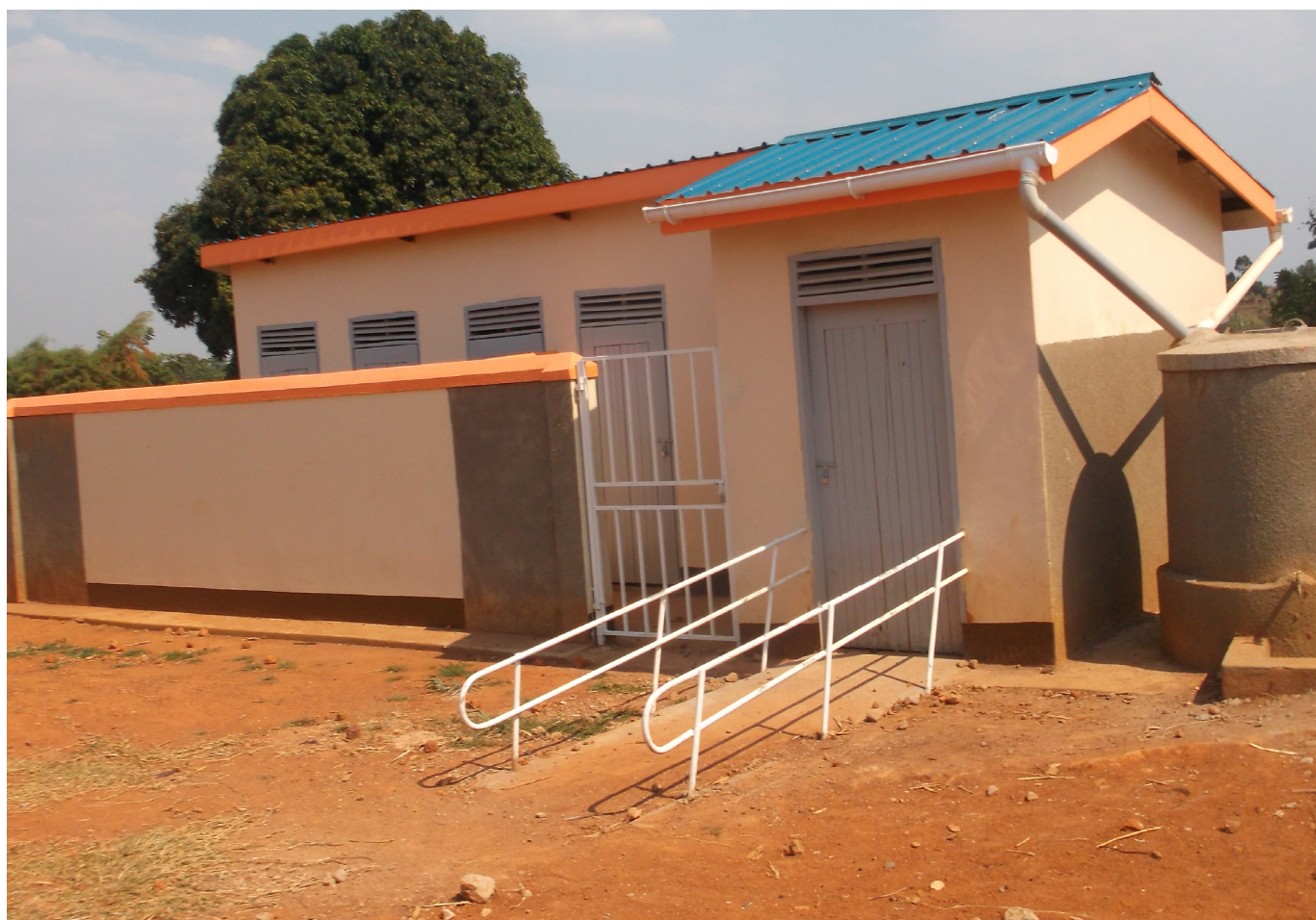
A school V.I.P latrine awaiting commissioning after completion of its construction. World Vision Uganda has constructed 16 such latrines, each with a special stance for children with disabilities
