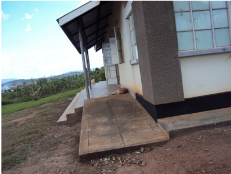
Ramp constructed at Health unit in Isingiro District
