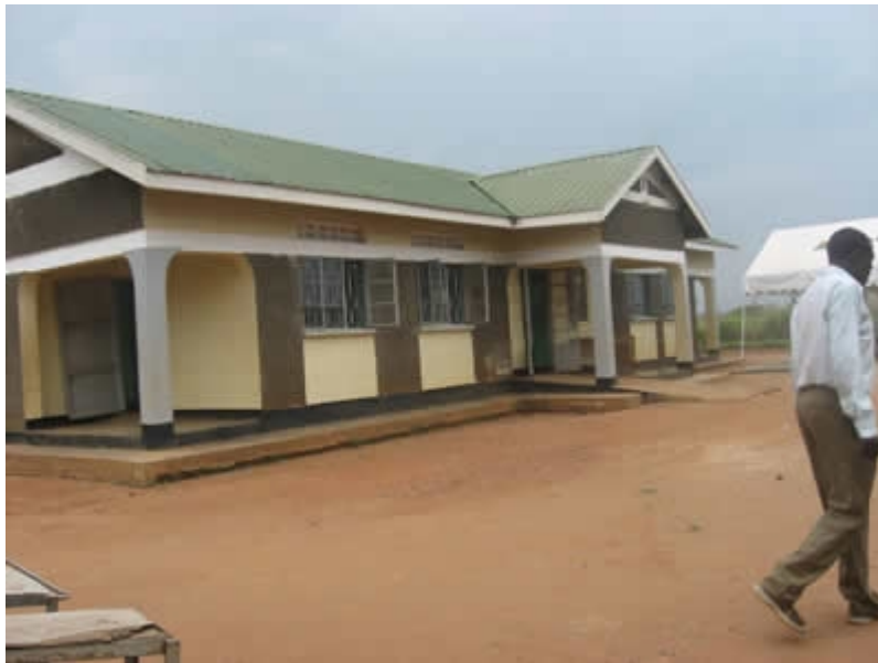
A ramp constructed at Bobi health centre 111-Gulu District.
